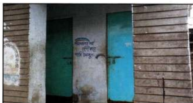
Figure 2: Renovated community latrine in Rupsha slum (2009), where community contribution was Tk. 1,455/= and ASEH grant was Tk. 7,029.
